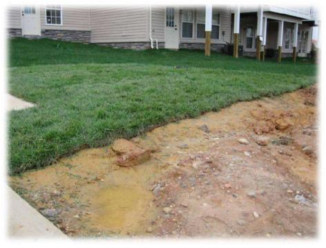
**Reduced Infiltration Rates** Increased soil strength & bulk density Decreased soil physical fertility Decreased water storage & supply Soil Impacts Reduced micro-organisms activities SOIL COMPACTION - 70 TO 99% REDUCTION Increased Stormwater Runoff Watershed Increased Flooding Impacts Decreased Water Quality **Reduced Channel Base Flow** Increased Stream Erosion
