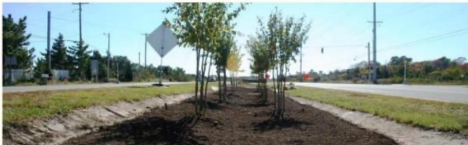
Storm water retrofits prevent water from washing into storm drains, allowing it to soak and filter into the ground
