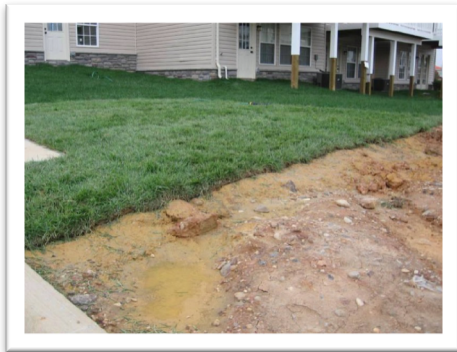
Figure 3 - Subsoils and Sod Installation in New Development (Source: Dr. Stu Schwartz)
