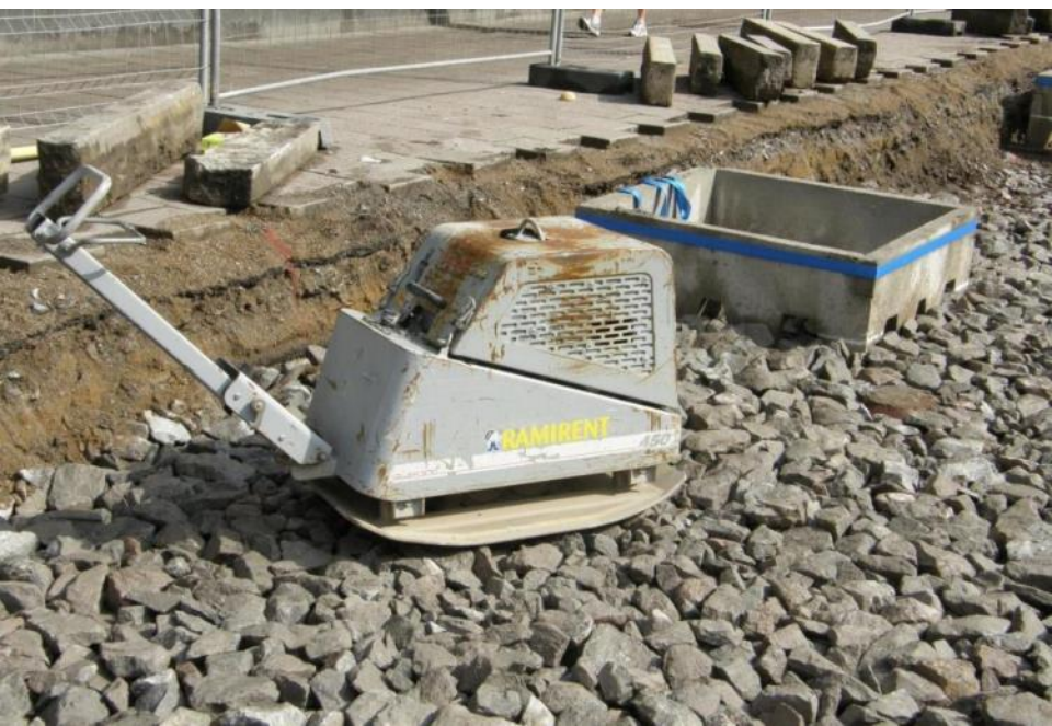
Compacting befor soil is washed in to the voids
