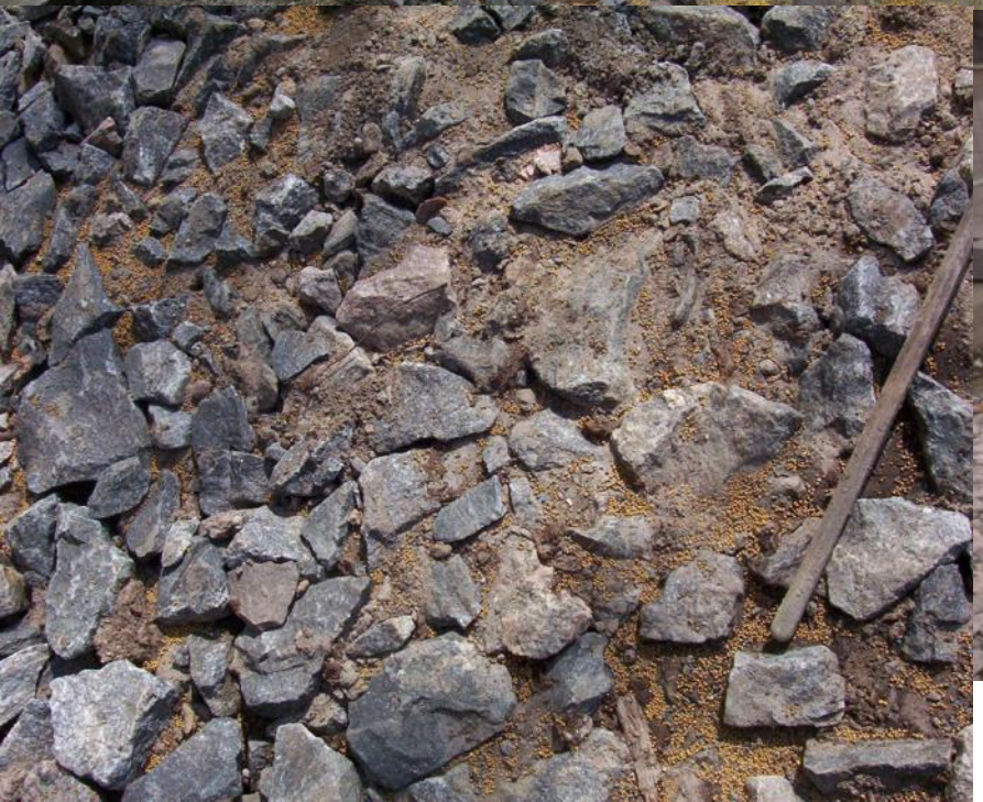
Layer for infiltration of rain water on top off the structural soil
