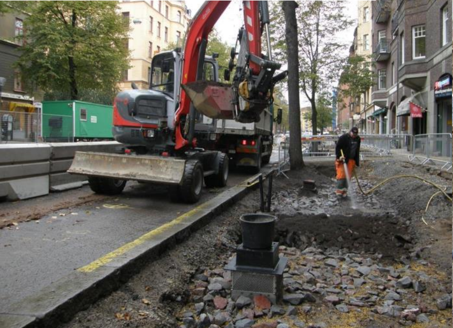
Flushing the soil into the structure
