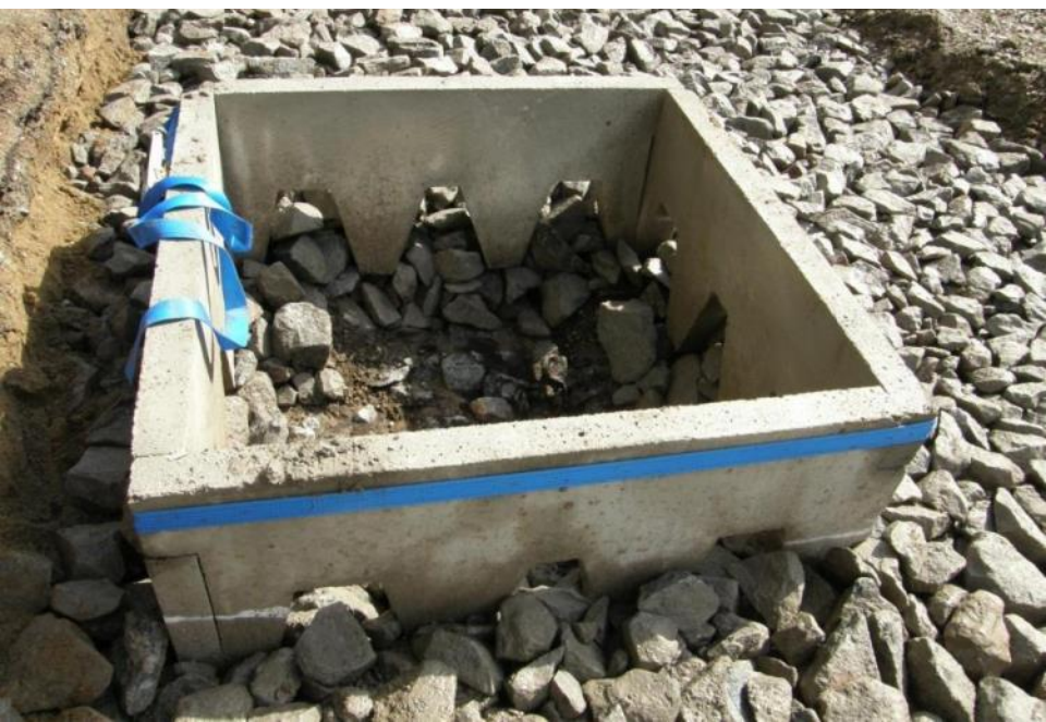
The stone shall fall into the box to get a stabel construction
