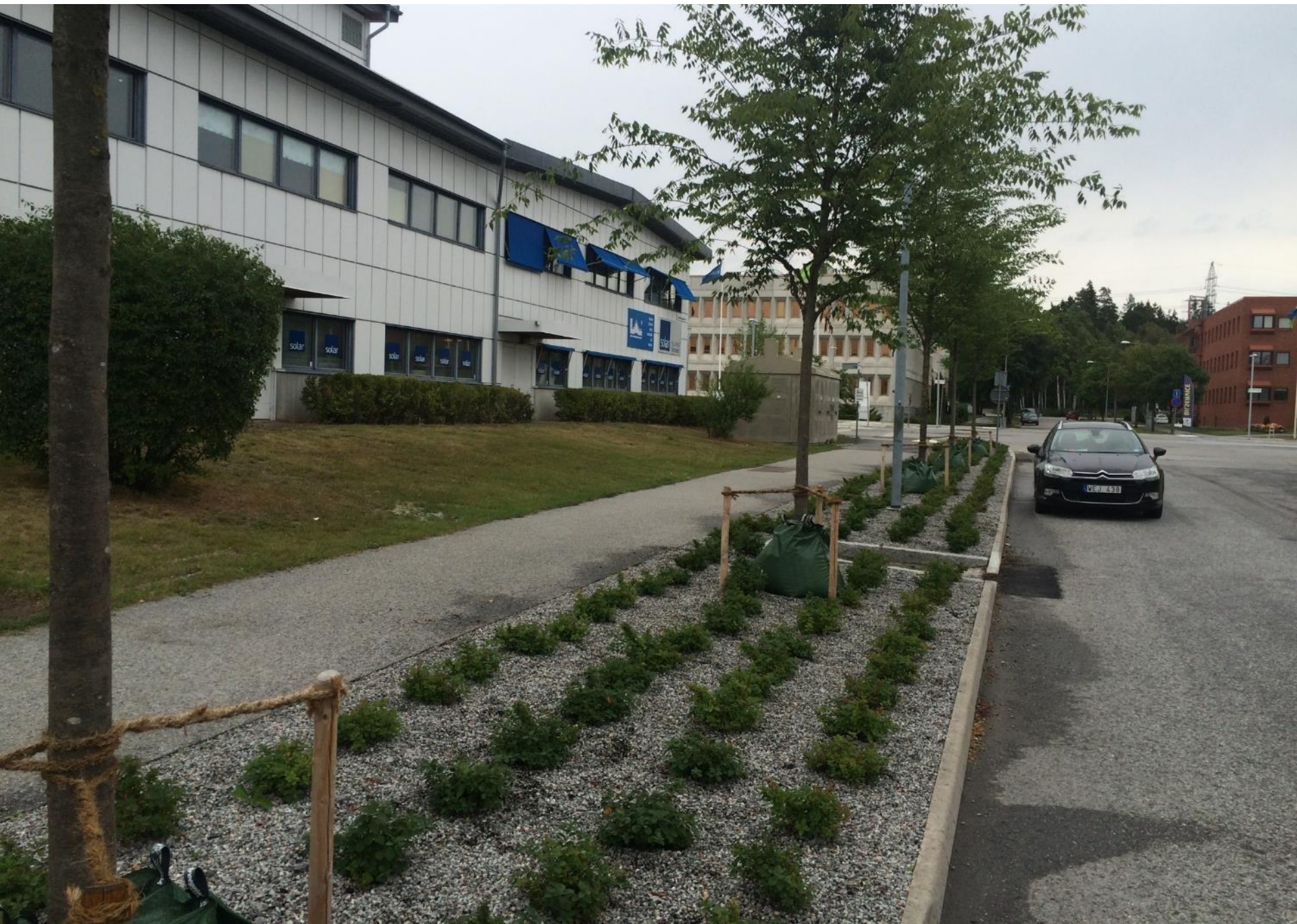
2017 Haukadalsgatan biochar 1 part, compost 1 part, macadam 4-8mm 6 parts
