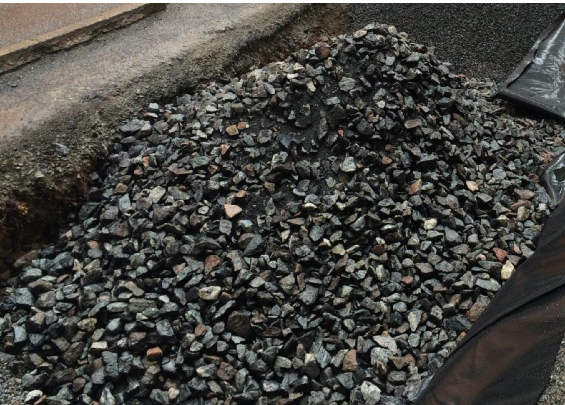
Biochar and stone chips = crushed granite (32-63 mm) and nutrient-enriched charcoal 15%. Volume premixed
